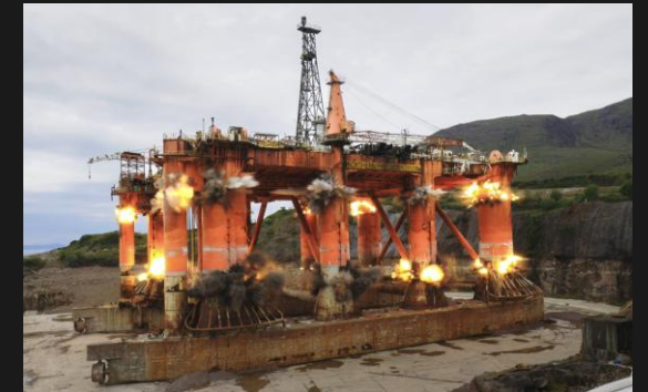
Onshore demolition & disposal
