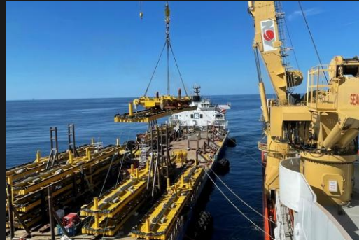
Offshore removal & transport
